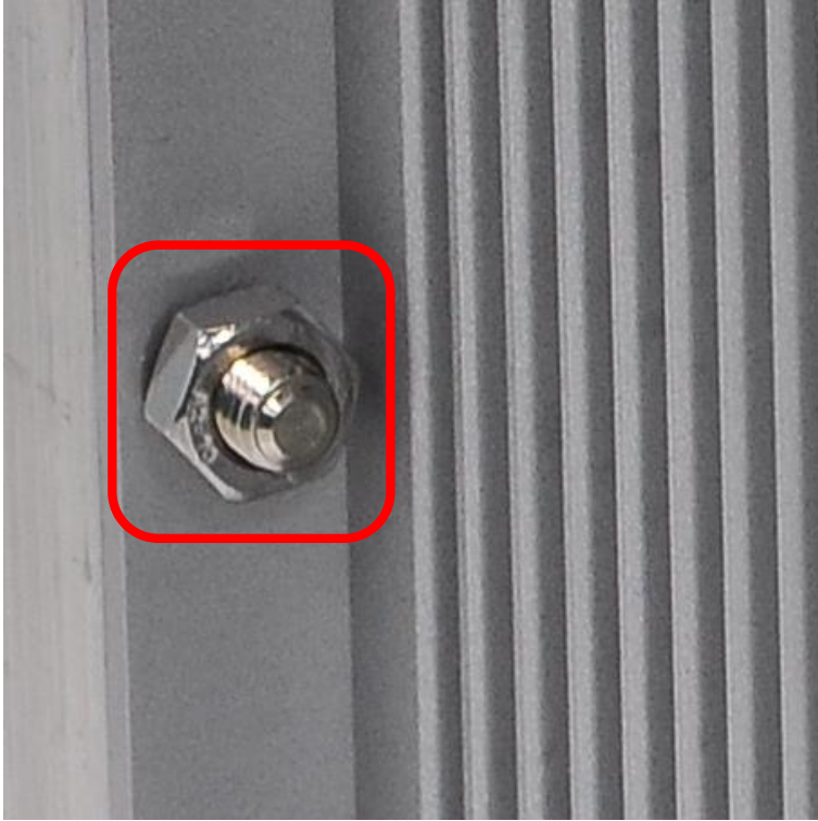
Ground screw of the switch
