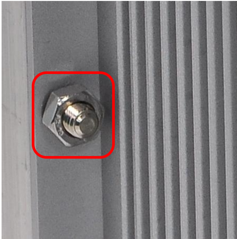
Ground screw of the switch
